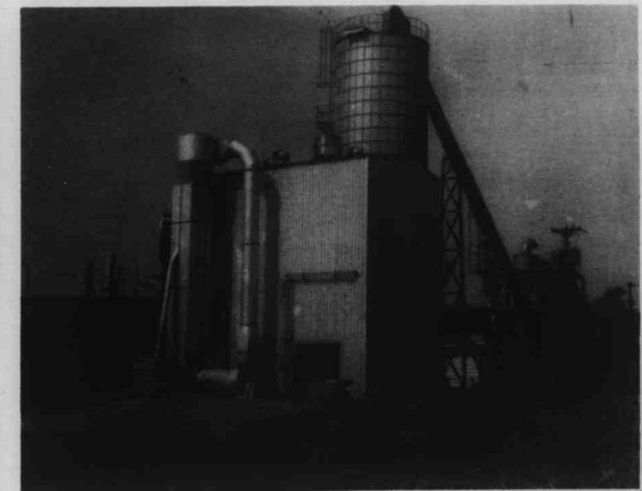
American Walnut Company received an SBA Air Pollution Control Loan to help finance this custom-designed woodburning boiler plant, which incinerates 45 tons per day of sawmill waste. It generates more than enough steam for the manufacturing plant and the drying kilns.
